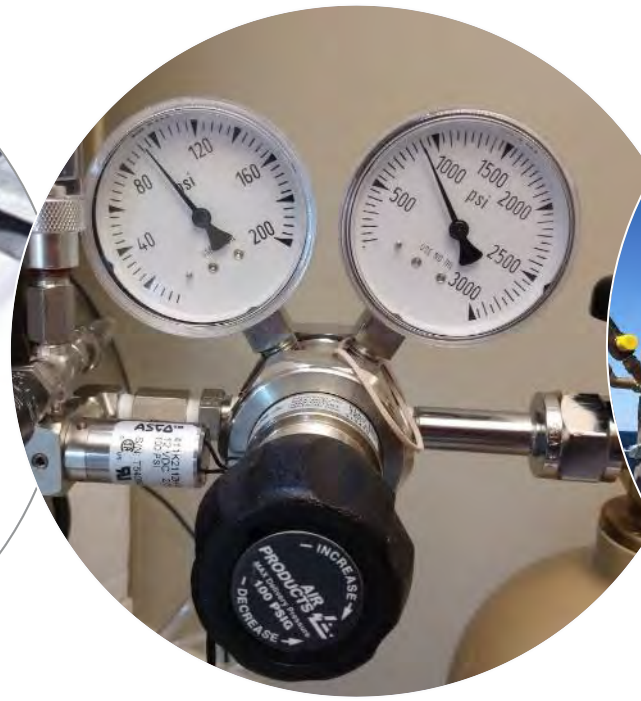
Pressure-test with dry nitrogen and evacuate.
