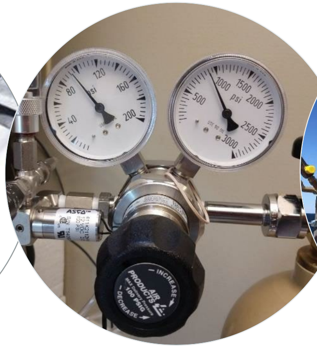
Pressure-test with dry nitrogen and evacuate.
