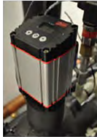
Flash Tank (Receiver)
